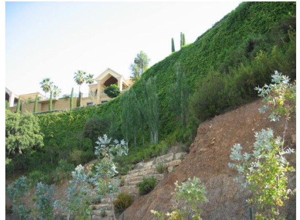
Figure 1 Fully vegetated TensarTech GreenSlope
