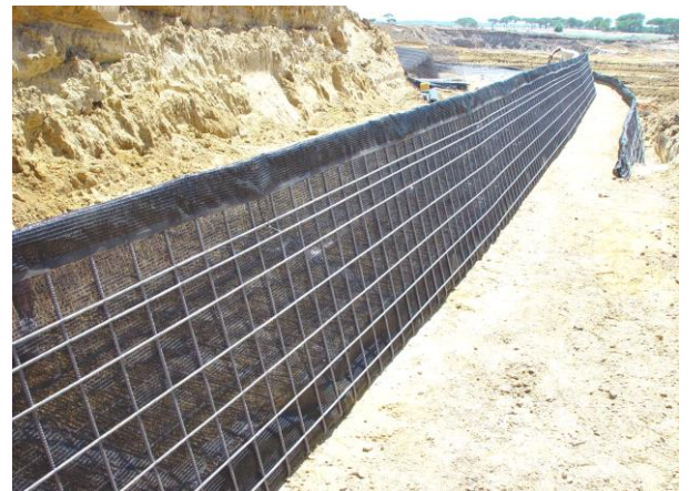
Figure 4 TensarTech GreenSlope facing panels in place prior to backfilling
